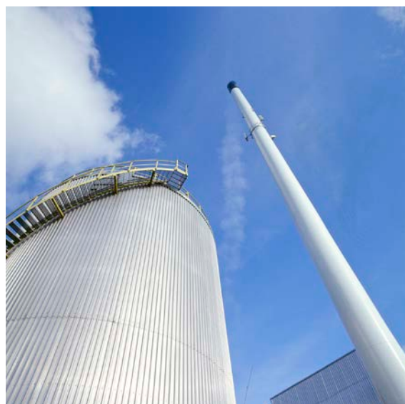
Incineration plant, Denmark
