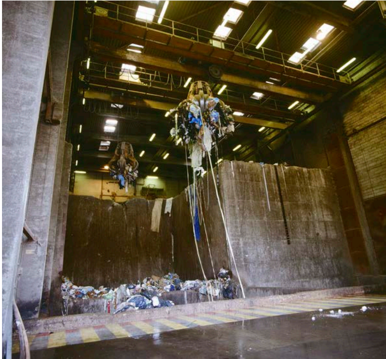
Incineration plant, Denmark
