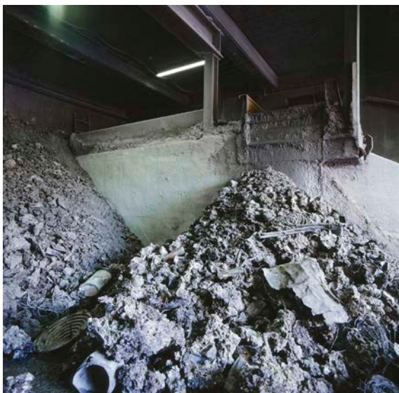
Incineration plant, Denmark
