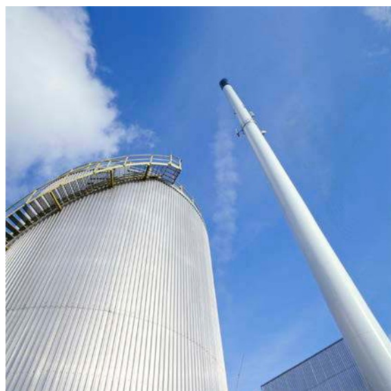
Incineration plant, Denmark
