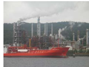
PVC plant, Norway
