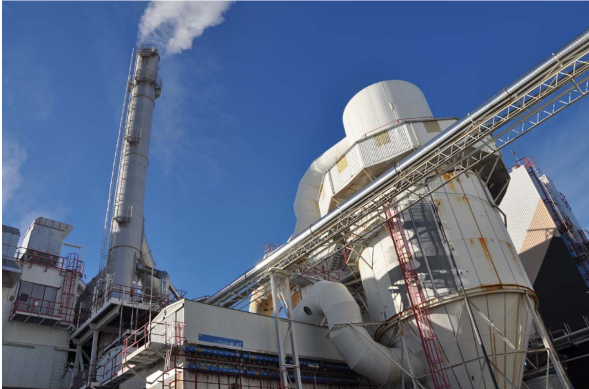
PVC plant, Sweden
