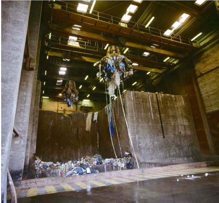
Incineration plant, Denmark
